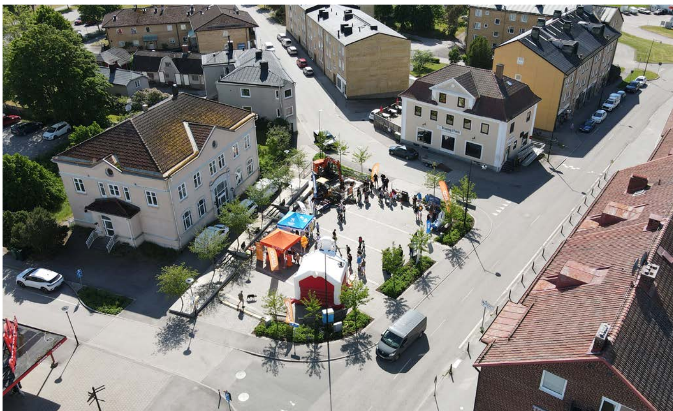
In Gullspång a new primary sub-station will enable electrification of industry and connections to renewable energy and charging infrastructure. In May, an information event was held for the general public, partners, and other stakeholders.
